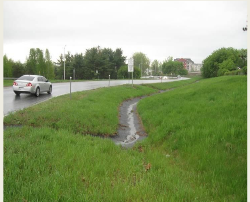
I-89 Exit 14 - enhancement needed to address paved swale
