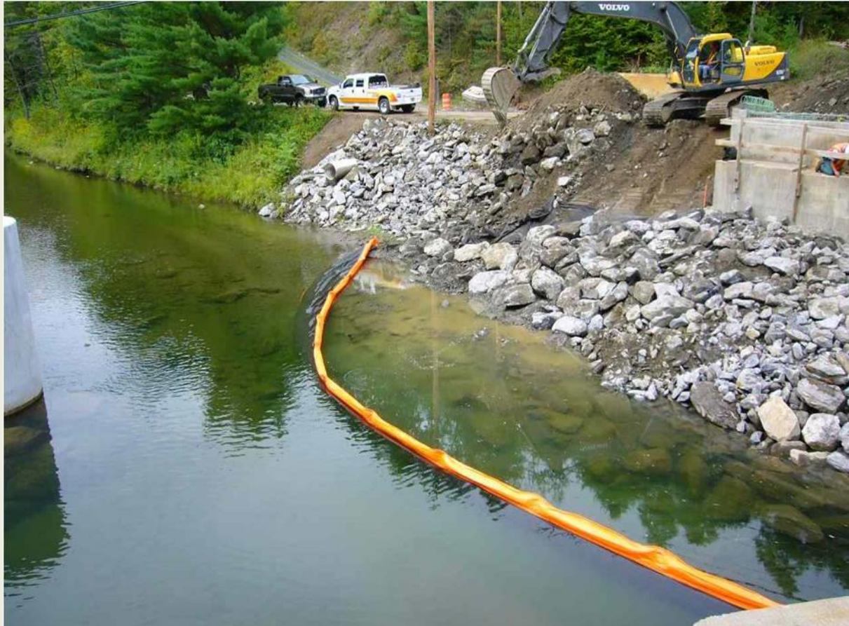
Filter curtain at work Rt. 110 Tunbridge, VT
