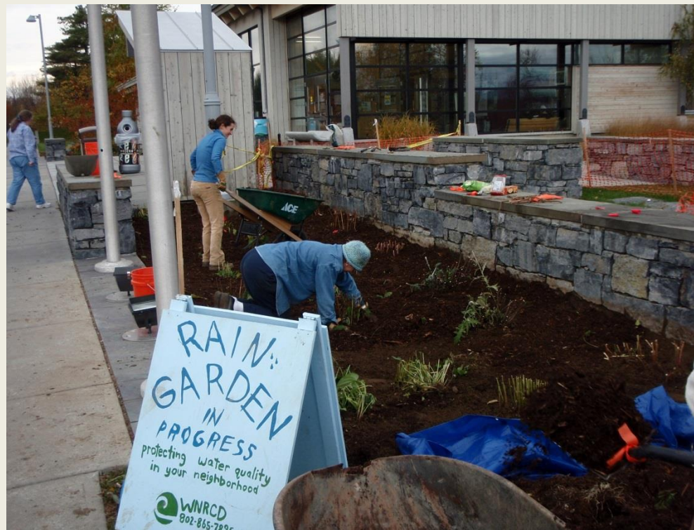
Williston I-89 NB Welcome Center Rain Garden Installation
